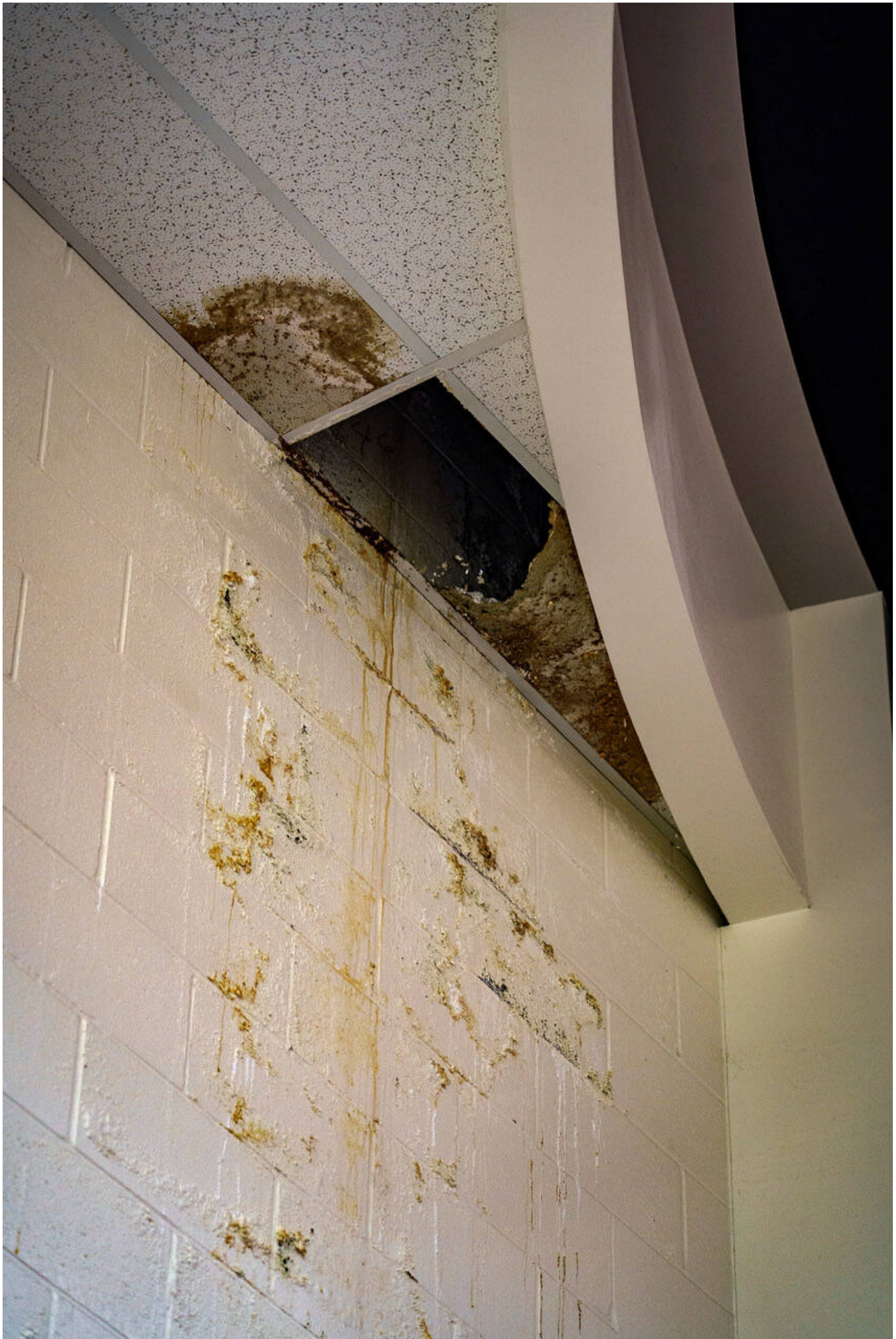
A gaping hole in the ceiling of a room near the auditorium points to excessive water damage. (Photo by David Welton)
